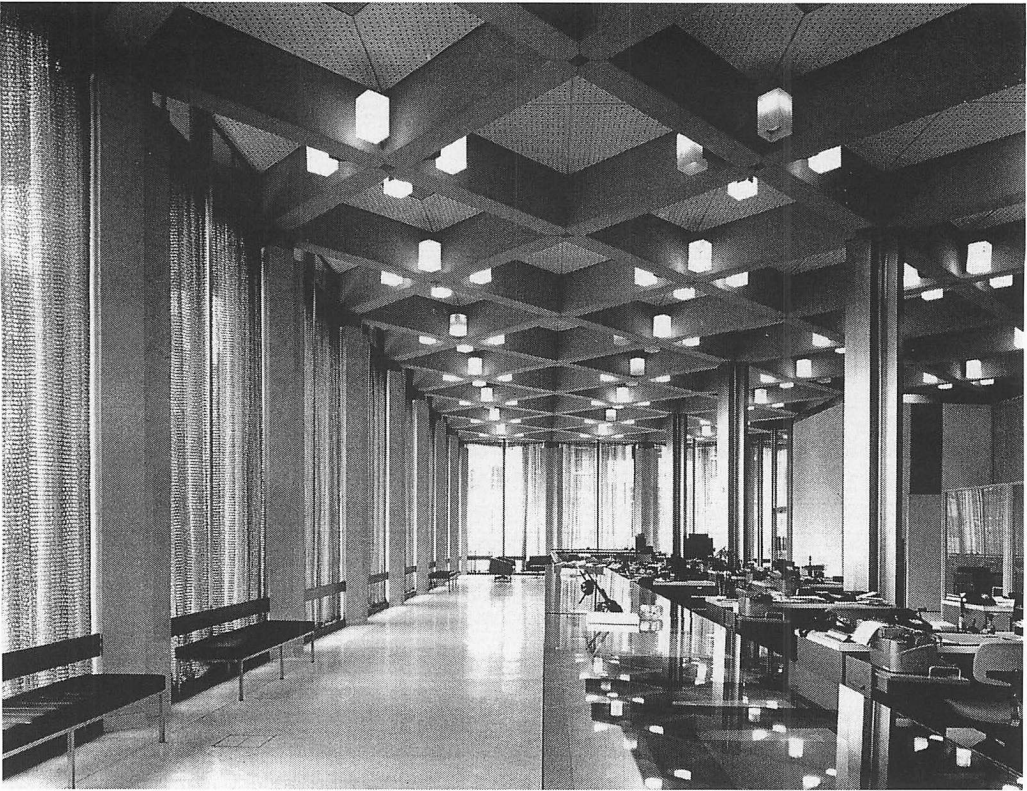
11. London, U.S. Embassy. Eero Saarinen (1956–60). Consular Section on first floor, with diagrid structural system above. Photograph copyright Balthazar Korab, 1960, from Library of Congress, Balthazar Korab Archive.
