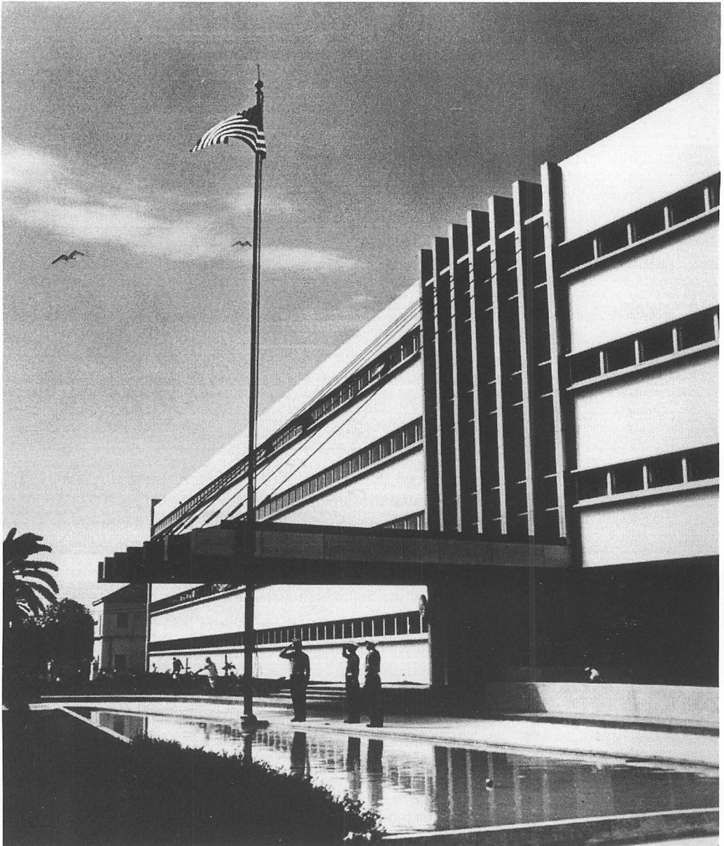
5. Karachi, former U.S. Consulate General, which had been the Embassy until 1960, when Pakistan's capital moved to Islamabad. Neutra & Alexander (1955–59). This building was decommissioned in 2011. Photograph courtesy U.S. Department of State.
