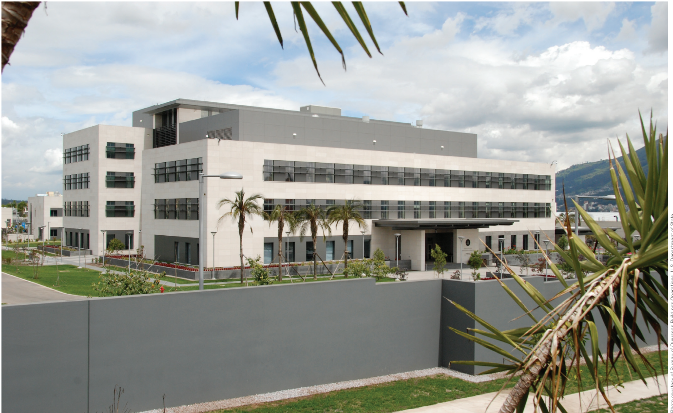
Photo courtesy of Bureau of Overseas Buildings Operations, U.S. Department of State
