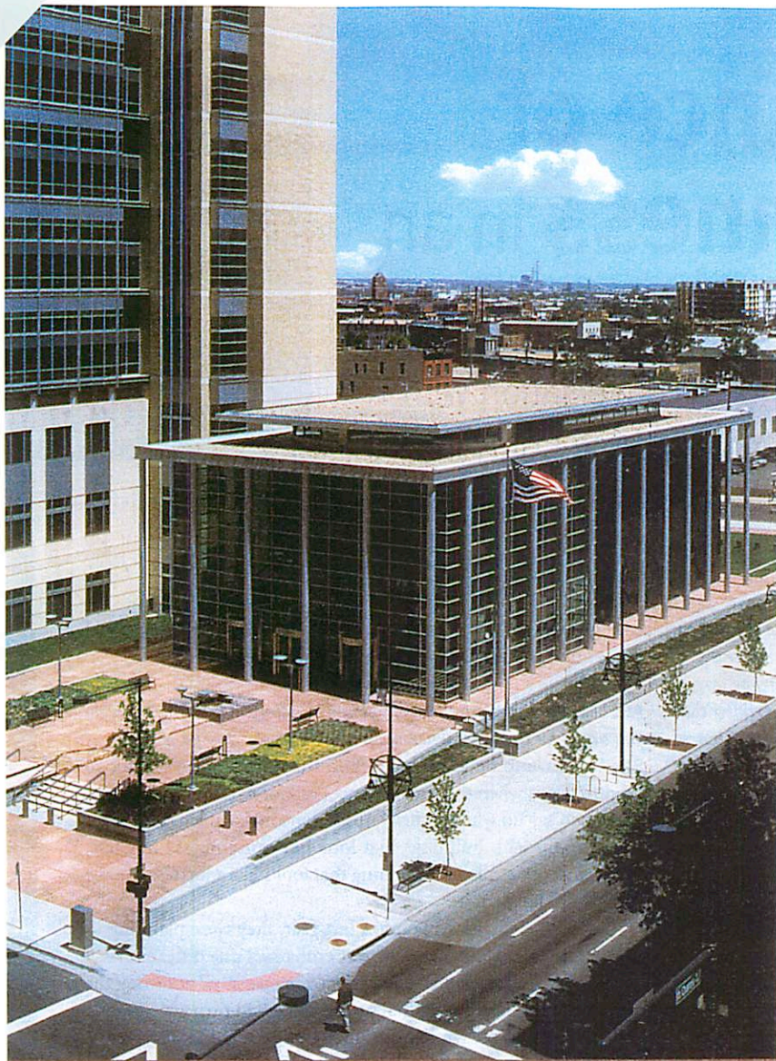
At the Arraj Courthouse, the plaza and lobby pavilion are publicly welcoming, yet discourage vehicle bombs and limit a terror attack's damaging effects.
