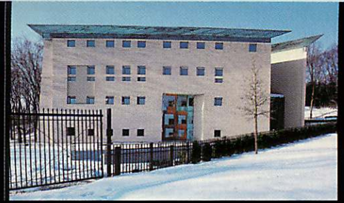
Italian embassy in Washington, D.C., by Piero Sartogo Architetti, with Leo A. Daly, photo: Robert H. Loeffler
