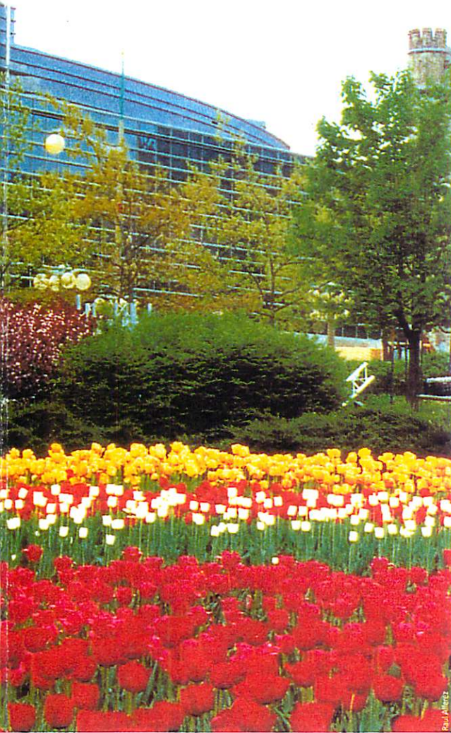
Above: West facade of the new American embassy in Ottawa. Architect David Childs headed the Skidmore, Owings & Merrill design team
